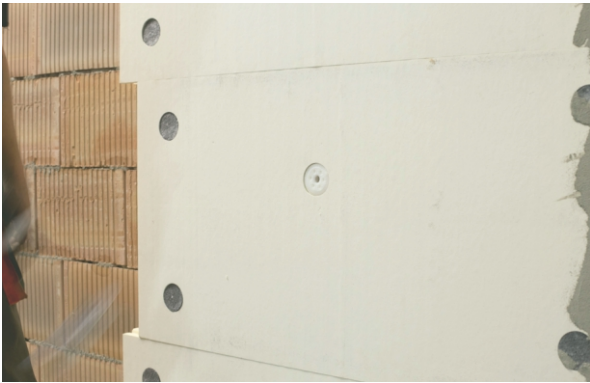
Figure 16. View of an anchor screw after installation
