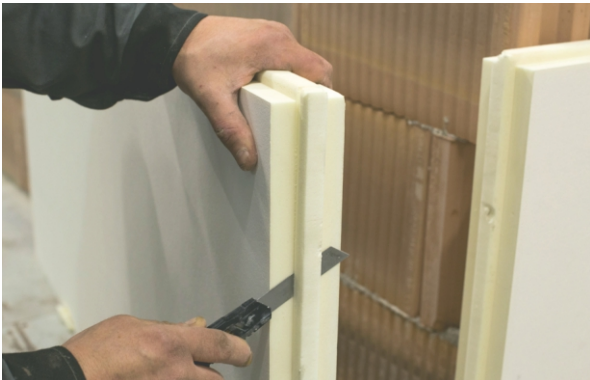
a) Cutting the tongue of the interlocking joint.
