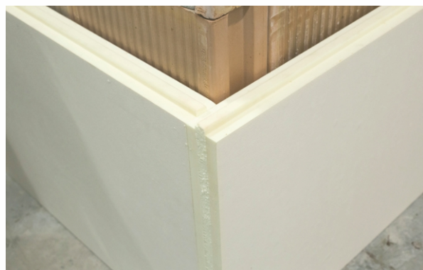
Figure 11. View of corner boards after installation
