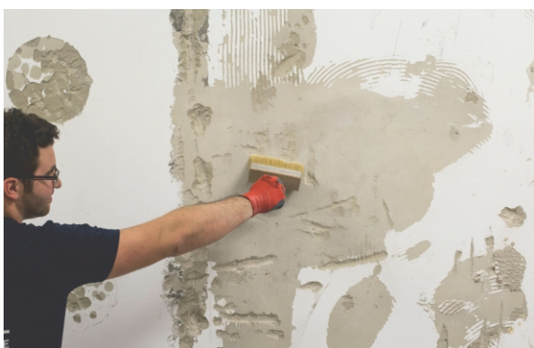
STAGE II Removing fine dust from the substrate
