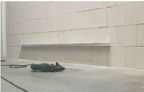
Figure 5. A properly installed starter strip
