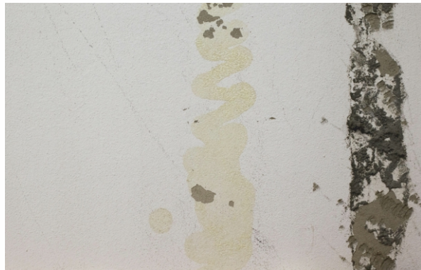
Figure 4. Spots that may reduce adhesion of the adhesive
