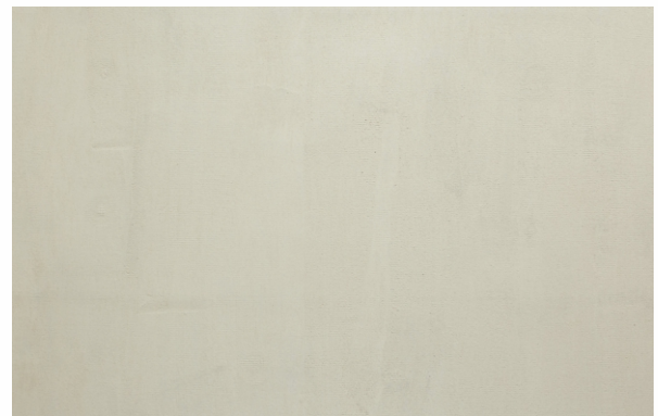
Figure 17. View of reinforcing layer after primer application
