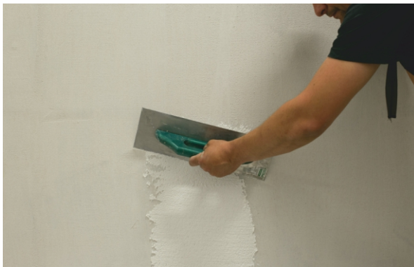
STAGE VI b) Installation of a finish layer
