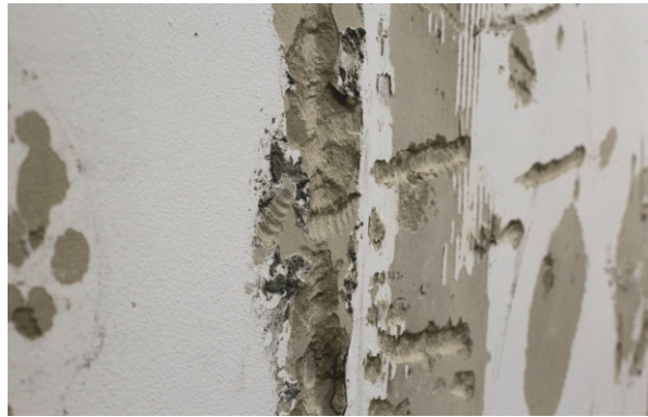
Figure 2. Matter remaining after previous finish layers were removed
