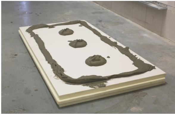
STAGE II. a) Distribution of adhesive on the board
