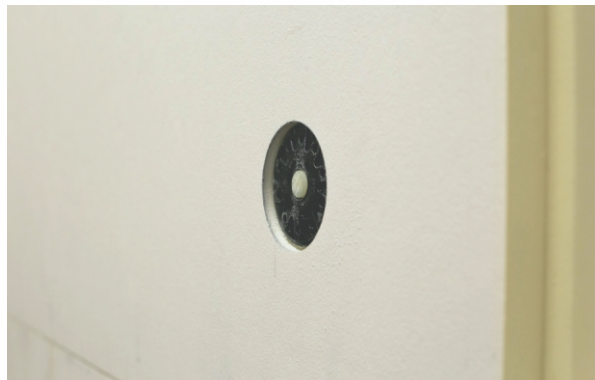
Figure 14. View of an anchor screw after installation
