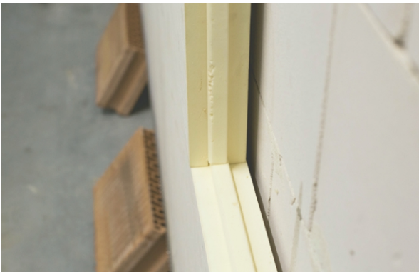
Figure 9. View of properly a positioned interlocking joint
