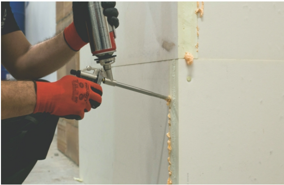
STAGE V a) Filling gaps with low pressure polyurethane foam.
