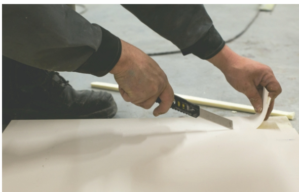
b) Removing the facing from the board section joined with the face of the lateral one.
