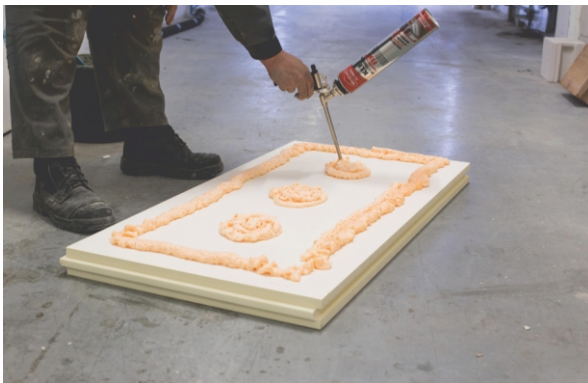
Figure 8. Distribution of polyurethane adhesive on the board
