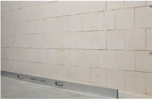
STAGE I. a) Determining the position of a starter strip
