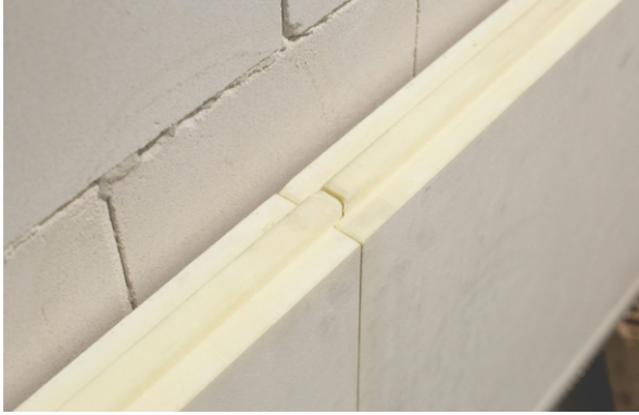
Figure 7. View of a properly positioned interlocking joint
