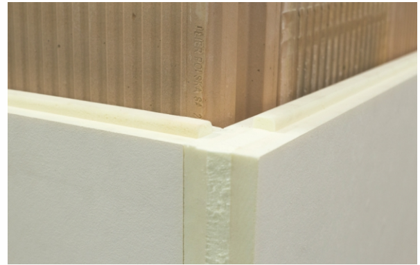
Figure 12. View of boards prepared for the installation of the next row
