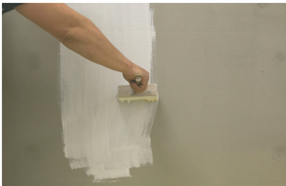
STAGE VI a) Priming of the reinforcing layer
