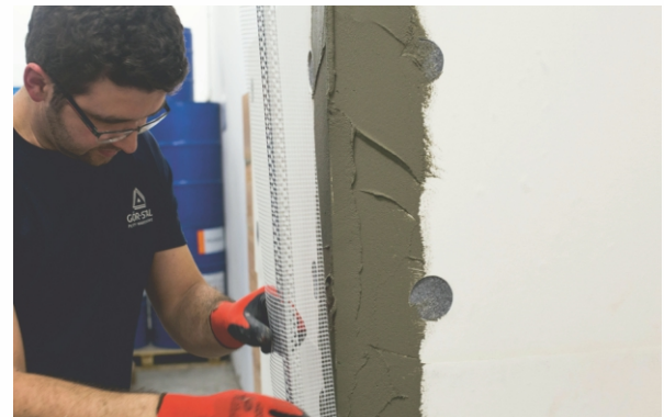
STAGE V c) Installation of a pre-made corner
