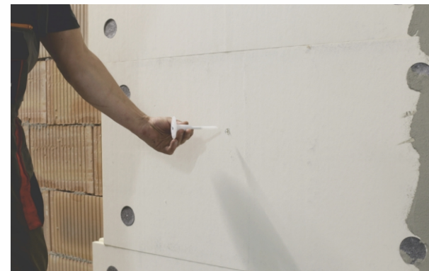
STAGE IV b) Embedding an anchor screw
