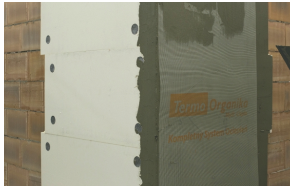
STAGE V e) Installing reinforcing mesh
