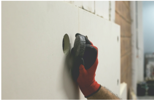
STAGE IV e) Installing a cap
