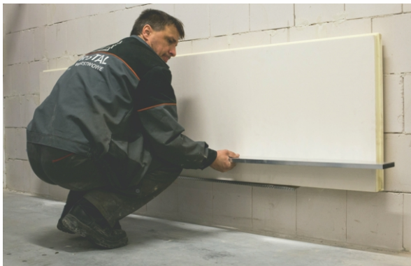
STAGE II. c) Installing and laying subsequent boards in the first row
