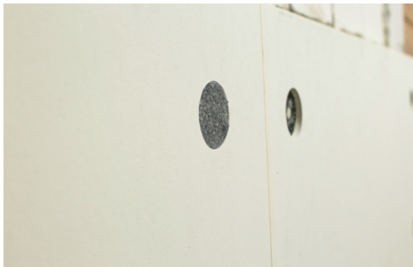
Figure 15. View of a cap after installation
