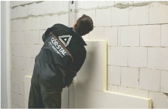
STAGE III a) Installing and positioning the second and third board rows
