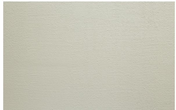
Figure 18. View of a completed finish layer
