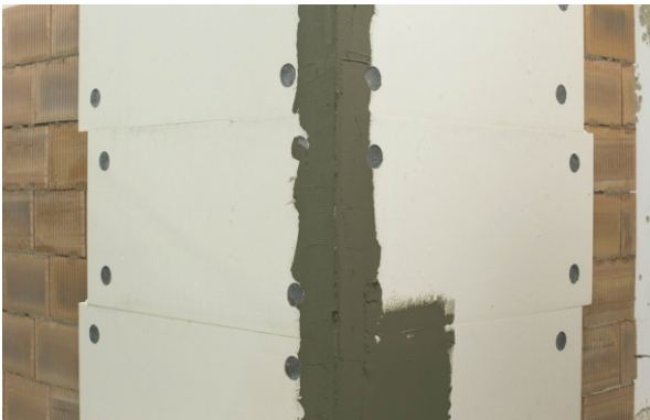
STAGE V d) Applying a layer of adhesive on the wall
