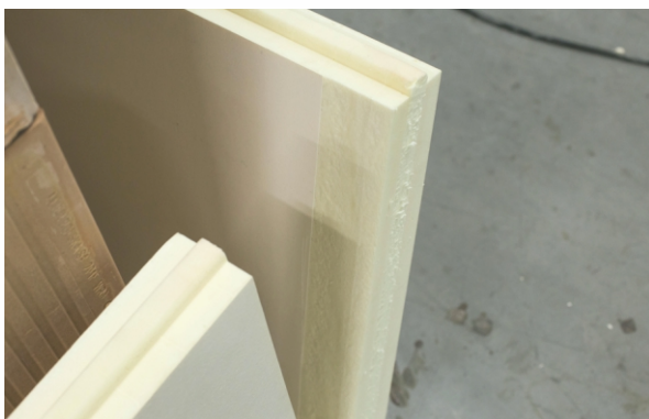
c) Installing corner boards
