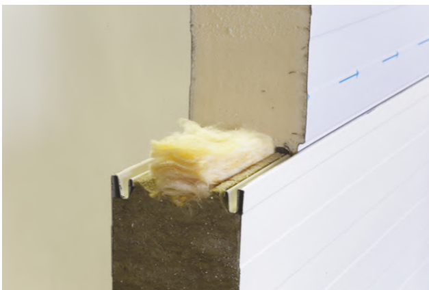
Photo. No. 2. View of the connection (overview)
